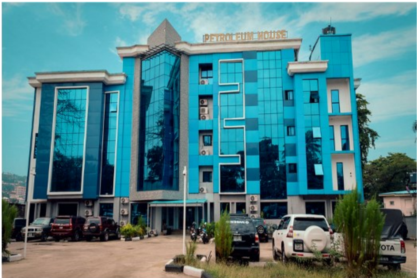
Petroleum Directorate Sierra Leone office Building
